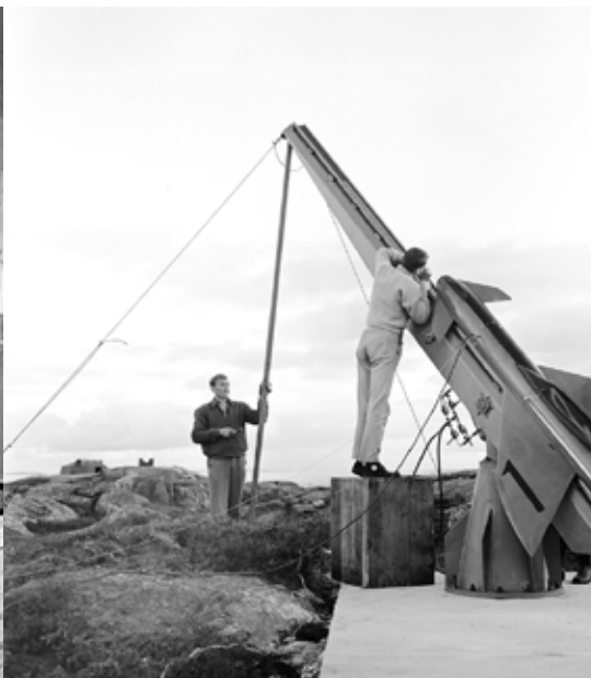
This photo from 1963 shows the very first Penguin missile, Enok, on the launch ramp. Its aerodynamic design had been tested in the wind tunnel, but this was the real deal.
